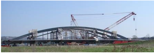
Figure 1. Construction of Dresden Bridge
